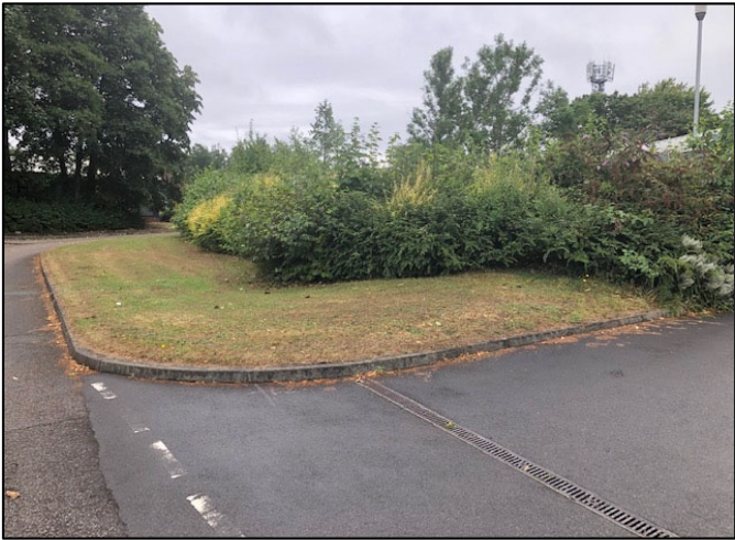
P22: SECTION 9, GENERAL VIEW
