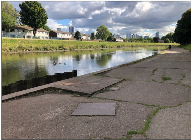
P32: SECTION 16 AND WIDER RIVER SECTION, VIEWED DOWNSTREAM
