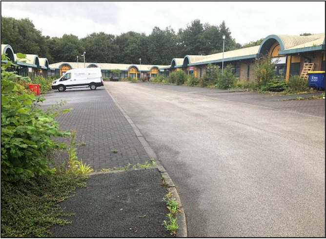
P21: SECTION 9, GENERAL VIEW
