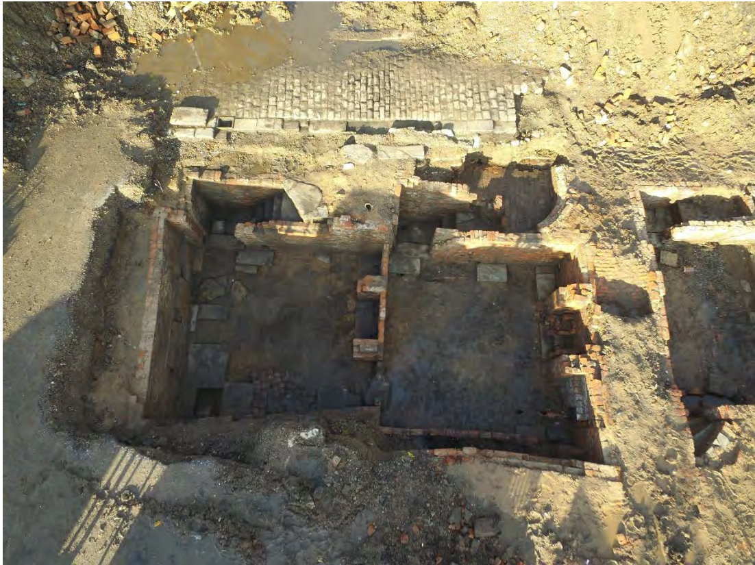
Plate 22: Building 4, north at top
