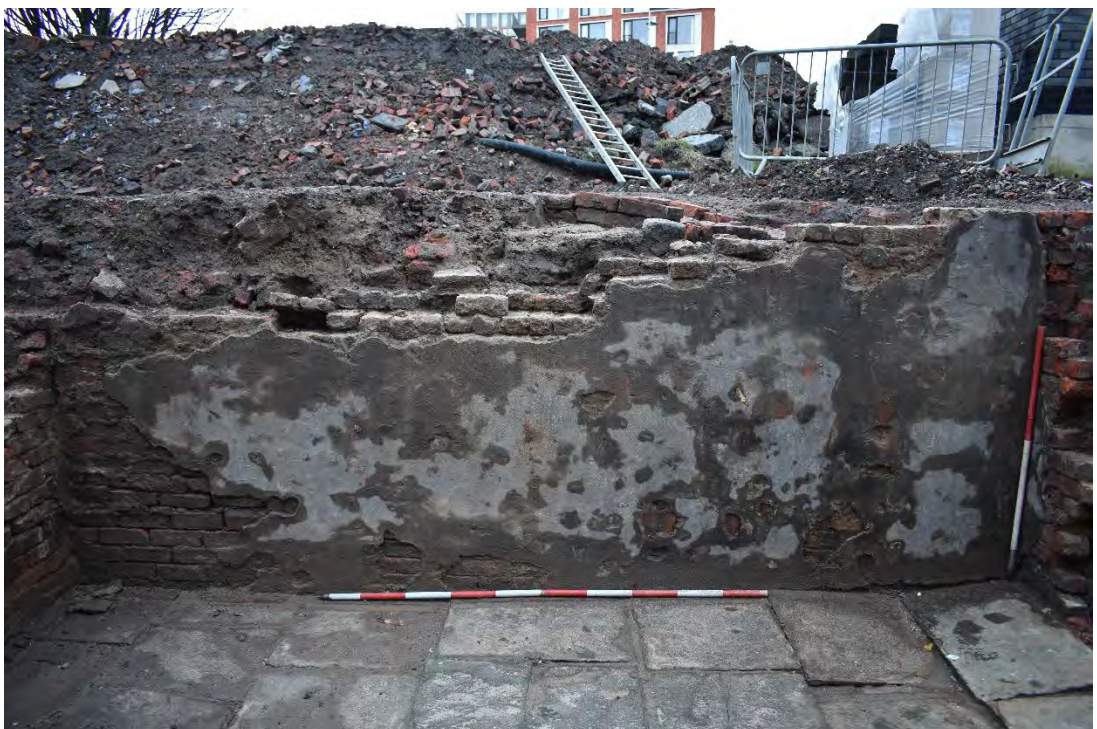
Plate 5: Cellar B, vertical scale against wall [05], looking west, scale: horizontal 2m, vertical 1m
