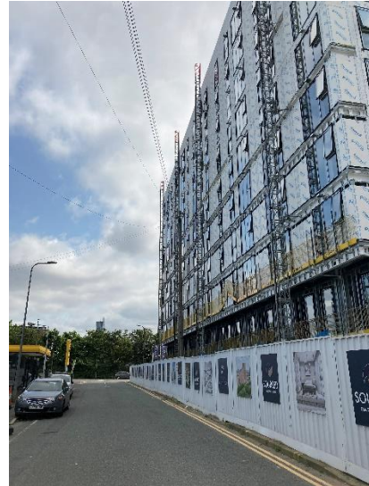
Figure 2.4: View from centre of Duncan Street looking east towards Oldfield Road, the City View construction site is in the right of the frame.
