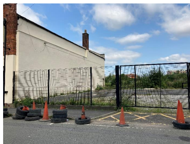
Figure 2.2: View of site from Duncan St, looking at the western party wall boundary.
