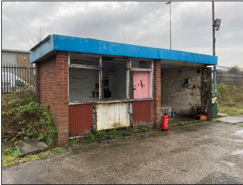
Photograph 10 showing the kiosk
