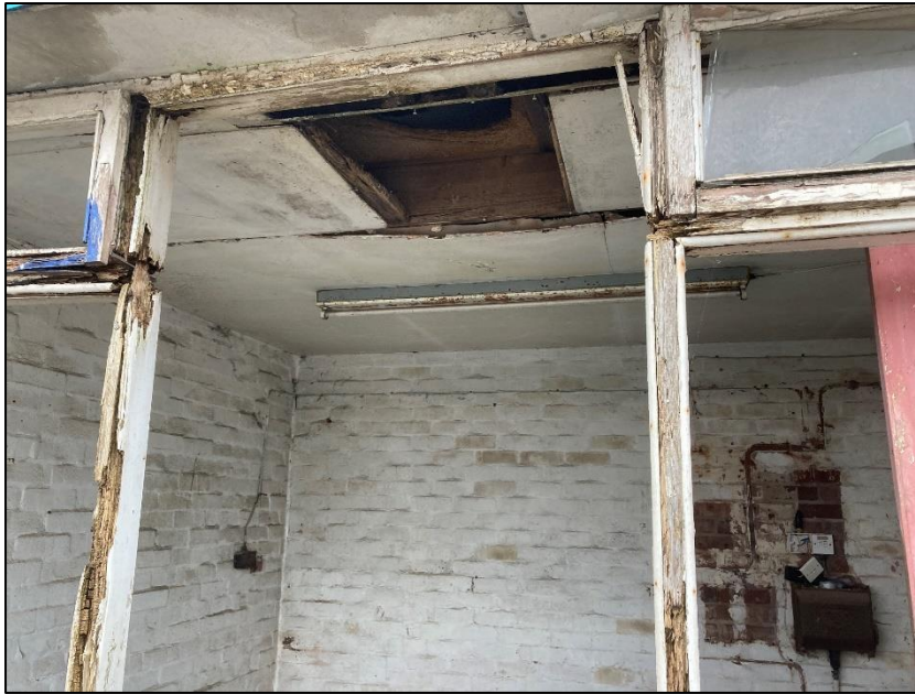
Photograph 12 showing the ceiling of the kiosk
