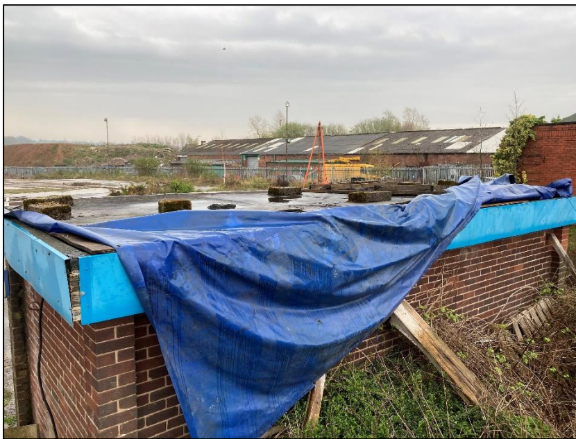
Photograph 11 showing the kiosk roof
