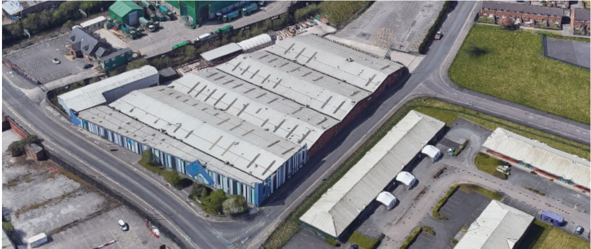
_Aerial View of Site (Looking from the East)
