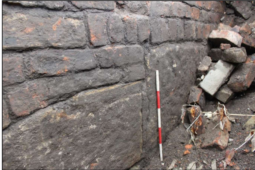
Plate 11: General shot of stone blocks [213] and [214], and brick wall [205], looking south-east. Scale = 1 x 0.5m.
