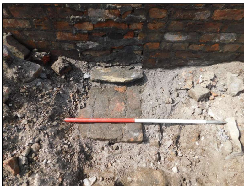
Plate 22: Shot of stanchion [113] and wall [107], looking south-west. Scale = 1 x 1m.
