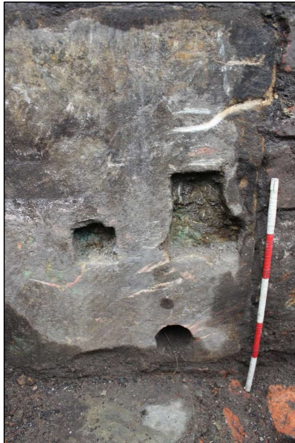
Plate 10: General shot of stone block [212] and brick wall [205], looking south-east. Scale = 1 x 0.5m.
