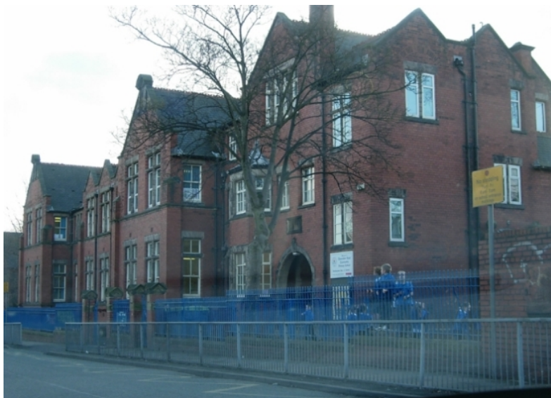
Clarendon Road Primary School, Clarendon Road
