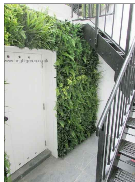
4: GREEN LIVING WALL WITH STEEL STAIRCASE
