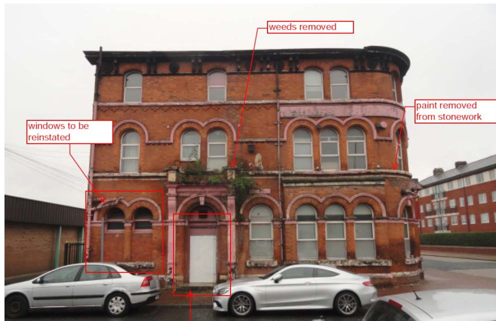
Proposed elevation works to Thurlow Street elevation
