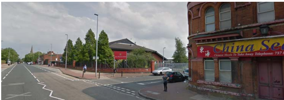
Army reserve building on the opposite side of Thurlow Road
