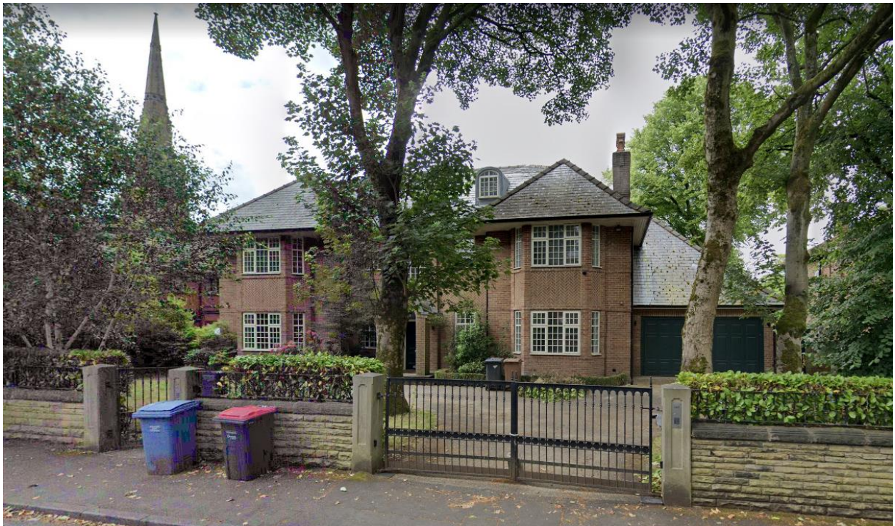
Similar large-scale development at no.27 Upper Park Road
