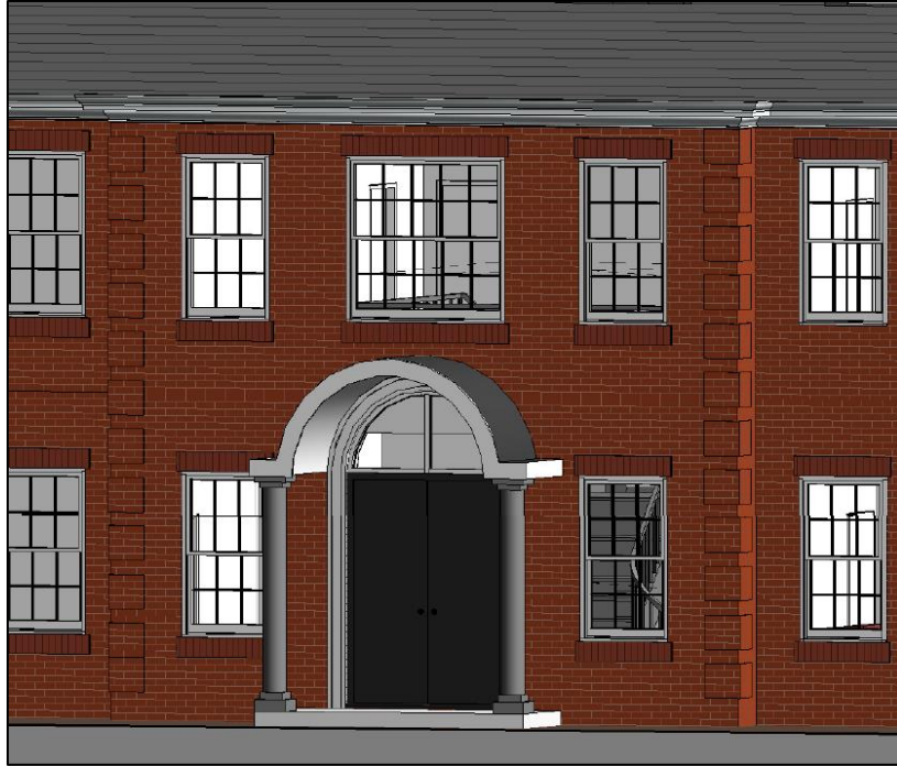
Magnified picture of front of property showing the protruding centre section of the front flank wall
