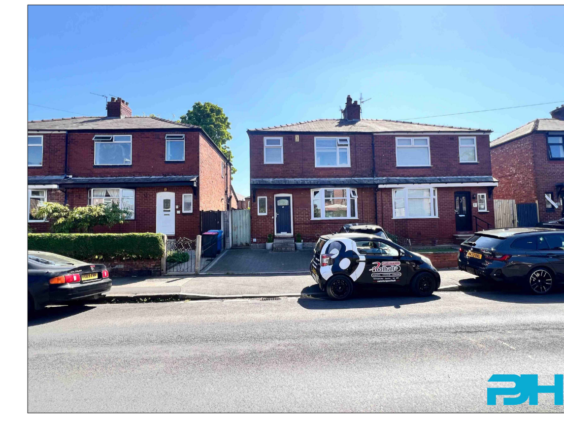
front elevation photo - Unaffected by proposed works
