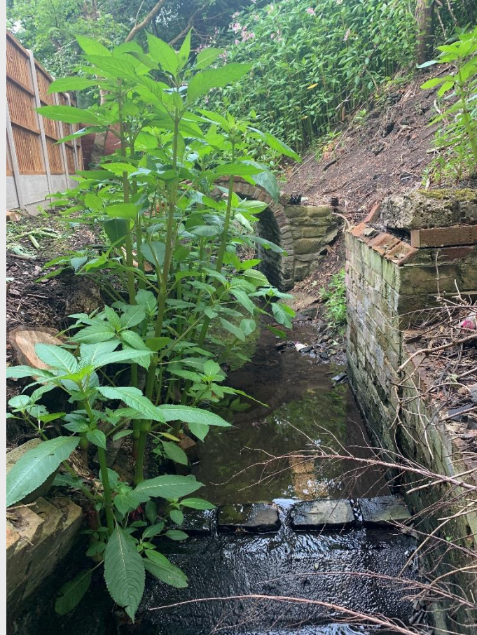
Photograph 8: Shaw Brook (West) with reinforcements
