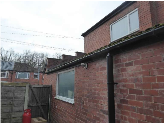
Side east elevation of garage with tight sealed fascias.
