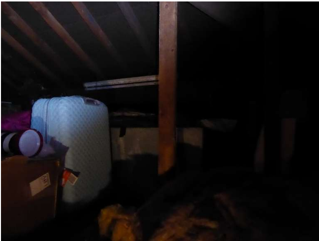
Cluttered loft space showing roof structure.
