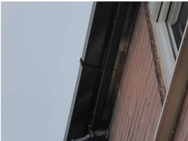
Front southern elevation with overhanging eaves sealed tight to brickwork.
