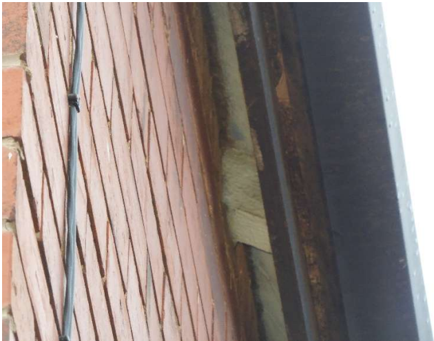
East side elevation with overhanging eaves sealed tight to brickwork.
