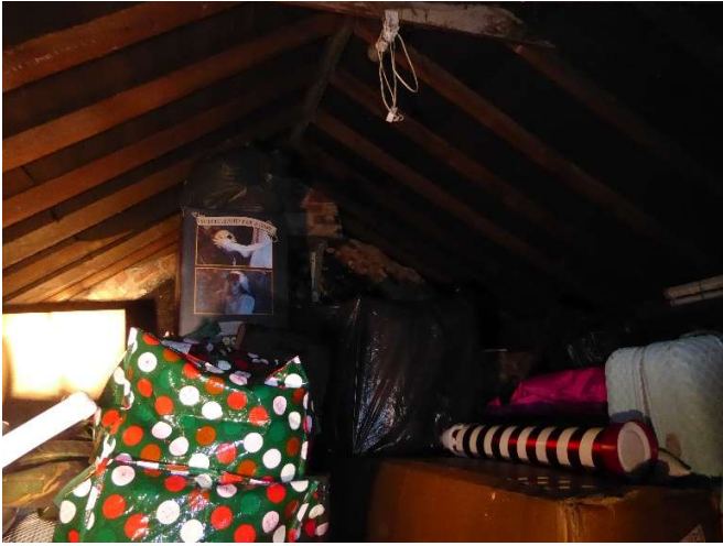
Cluttered loft space showing roof structure.
