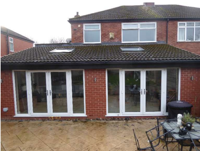
Rear elevation showing extension and tight sealed concrete tiles.
