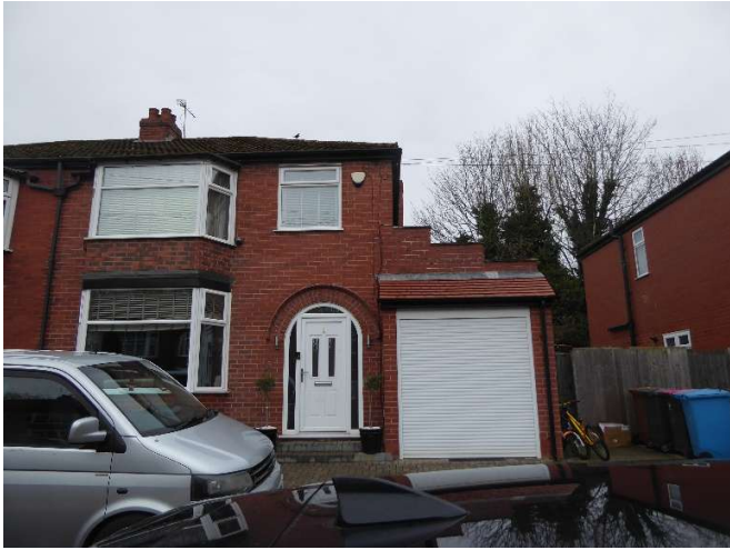
Front southern elevation, general view.
