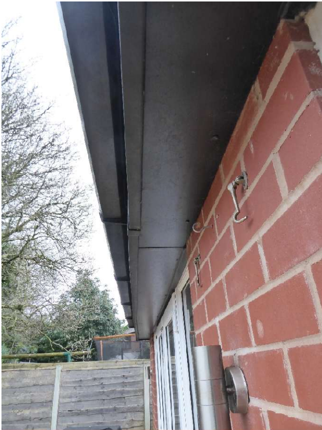
Rear elevation showing soffits tight sealed against brickwork.
