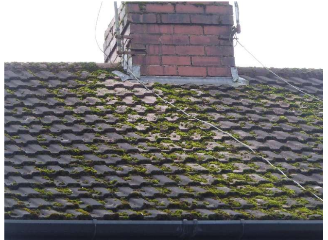
Rear elevation showing main roof and tight sealed concrete tiles.
