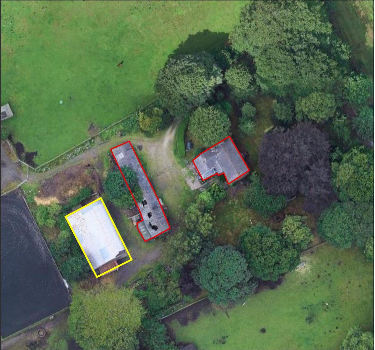
Figure 1.1: Aerial image of buildings at Olive Mount Farm, Irlam.
